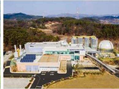
Biogas production facilities from food waste/food industrial effluents, Daejeon [Plant] Total Ground Area 6,016m 2 , Process Amount 400t/day
