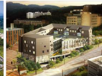
Convergence Science Center, Cluster Center, and Dormitory, Daejeon University [Education/Research Facility] Total Ground Area 27,191㎡, B1-9F
