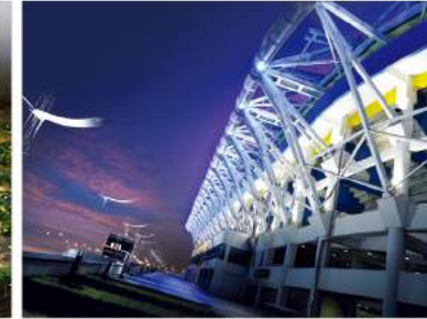
Daejeon World Cup Stadium [Sports Facility] Total Ground Area 100,597m 2 , B1-5F
