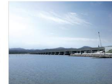
Chonamdaegyo Bridge [Bridge]
