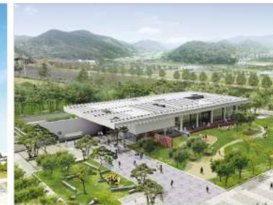
Lee Ungno Museum [Culture Facility] Total Ground Area 1,703m 2 , B1-2F, White Concrete Construction
