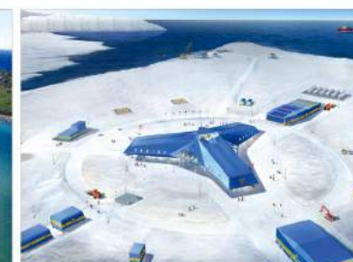
ANTARCTICA Jangbogo Station(Second Antartic Base), Antarctica Terra Nova Bay, Victoria Land, East Antarctica, Total Area 4,458m 2 , 16 Buildings, 24 Facilities/Equipment
