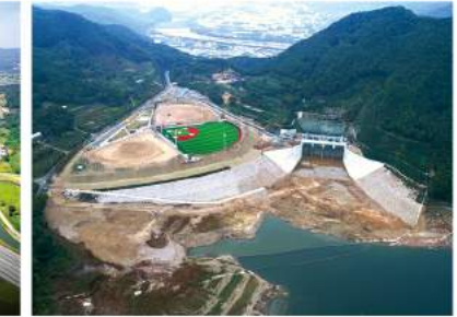
Unmun Dam Emergency Spillway [Agricultural Civil Works] Tunnel Type Spillway, Maximum Discharge 6,910㎡/s
