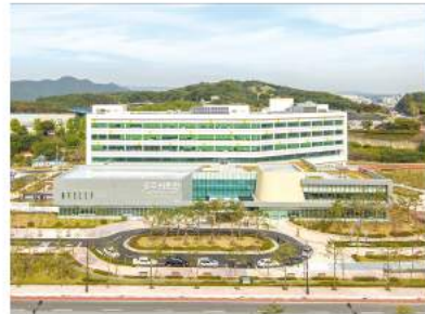
Gongju Medical Center [Medical Facility] Total Ground Area 31,538㎡, B2-6F, 361 Beds
