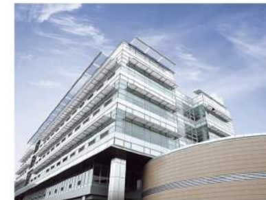
Nuclear Environment Technology Institute [Education/Research Facility] Total Ground Area 27,278㎡, B1-5F
