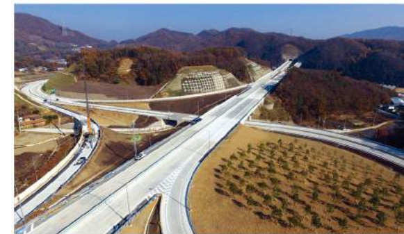
Yeongdong 2 (Gwangju-Wonju) Road Management Office Length 56.95km (4 Roundtrip Lanes) 5 ICs, 3 JCTs, 7 Operation Offices
