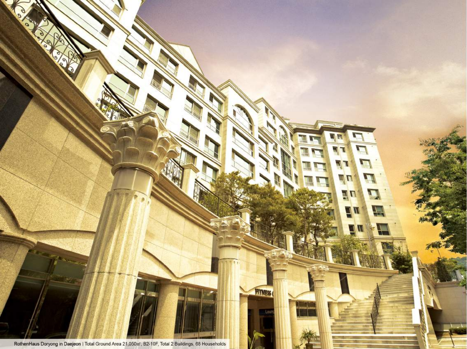
RothenHaus Doryong in Daejeon | Total Ground Area 21,050㎡, B2-10F, Total 2 Buildings, 68 Households
