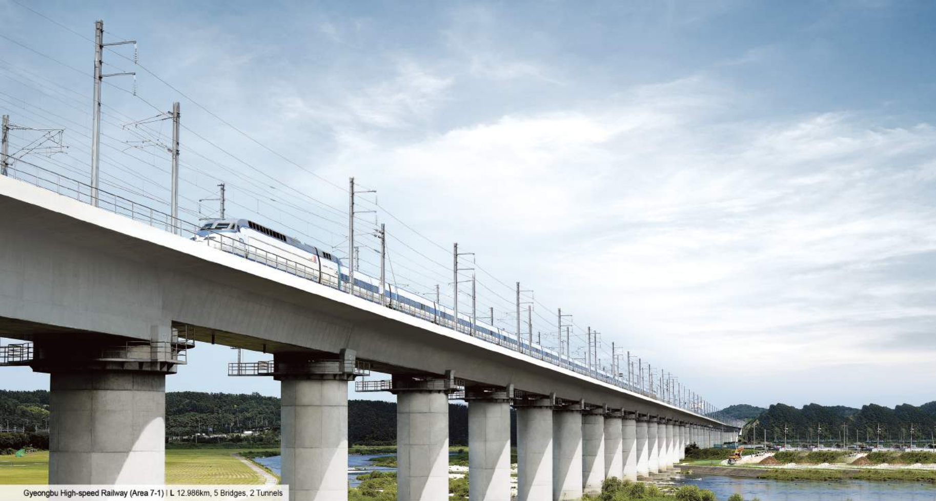
Gyeongbu High-speed Railway (Area 7-1) | L 12.986km, 5 Bridges, 2 Tunnels
