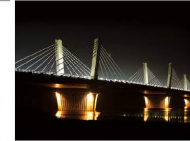
Daehodaegyo Bridge [Bridge]
