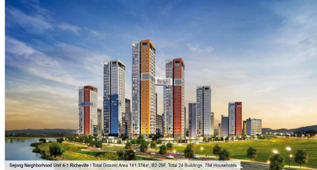
Sejong Neighborhood Unit 4-1 Richeville | Total Ground Area 141,374㎡, B2-29F, Total 24 Buildings, 784 Households
