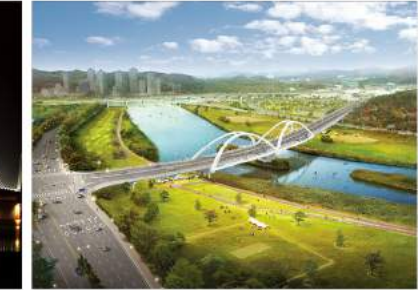
Hansaemdaegyo Bridge [Bridge]
