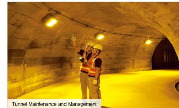
Tunnel Maintenance and Management
