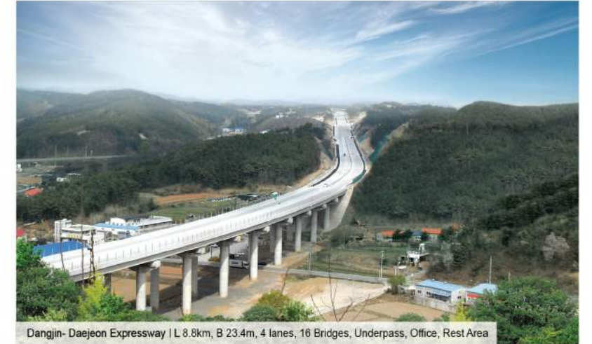
Dangjin- Daejeon Expressway | L 8.8km, B 23.4m, 4 lanes, 16 Bridges, Underpass, Office, Rest Area
