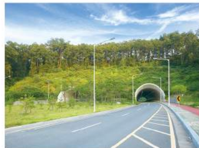
Yongun Tunnel [Tunnel] L 1.572km, B 25m, 4 Lanes
