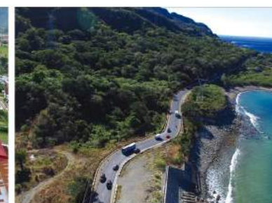
PHILIPPINES PBM-1 Road Project Section 1 / Section 2 Middle/North Luzon Island, Philippines Section 1: L 146km, Section 2: L 96km
