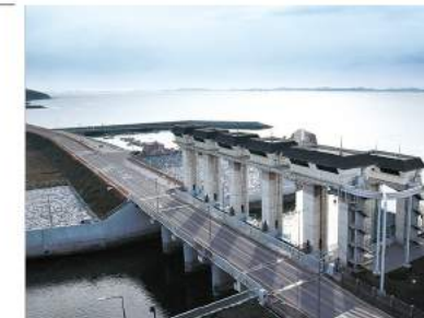
Hongbo District Agricultural Development Project [Agricultural Civil Works] Breakwater(L 1,865m, B 16.1m), Tidal Gate(118㎡) Bridge(59.6m), Entrance Road(L 10.212km, B 9m), Miter Gate
