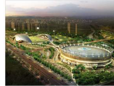
Incheon Namdong Asiad Stadium [Sports Facility] Total Ground Area 42,356m 2 , B2-3F, Seating Capacity 13,535(Gymnastics Stadium, Rugby Field)
