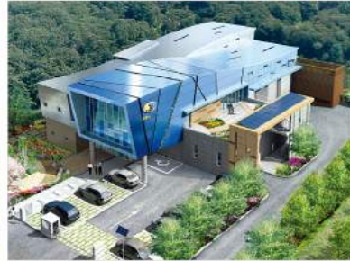
Auto Clean Net in Hangang New Town, Gimpo [Plant] Total Ground Area 5,586m 2 , Processed Amount 77.35t/day
