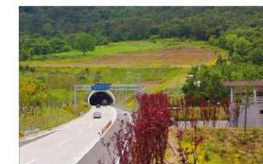
Boseong Branch Tunnel Comprehensive Center 7 Long Tunnels, 28 Short Tunnels
