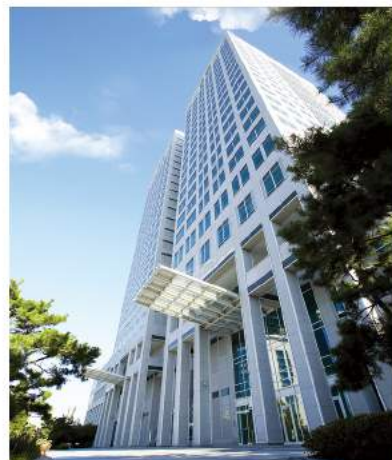
Daejeon City Hall [Office Facility] Total Ground Area 87,213㎡, B2-21F
