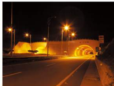
Galsan Tunnel [Tunnel] L 770m (Northbound 375m, Southbound 395m), B 7.85m, 2 Lanes
