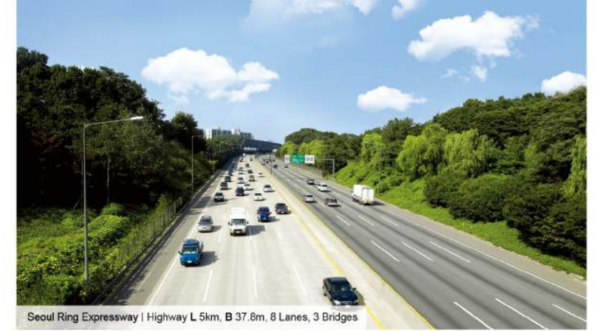
Seoul Ring Expressway | Highway L 5km, B 37.6m, 8 Lanes, 3 Bridges
