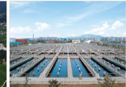
Daejeon Sewage Treatment Facility [Environment Facility]
