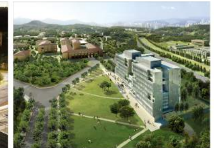
Kim Byung Ho IT Convergence Center, KAIST [Education/Research Facility] Total Ground Area 25,464㎡, B1-10F
