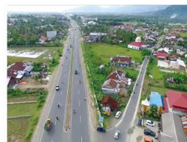
INDONESIA Padang Bypass Expansion Project, Indonesia Indonesia Sumatra Island Padang City L 27km, Road Expansion(2 Lanes → 4 Lanes)
