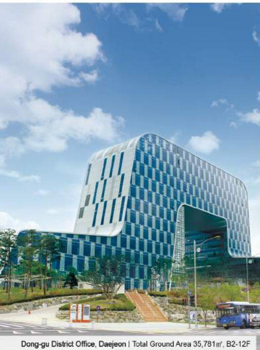
Dong-gu District Office, Daejeon | Total Ground Area 35,781㎡, B2-12F
