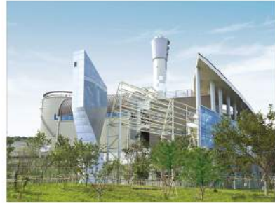
Community Energy Facilities in Southwestern Daejeon [Plant] Total Ground Area 12,823m 2 , Steam Turbine Generation 48.3MW
