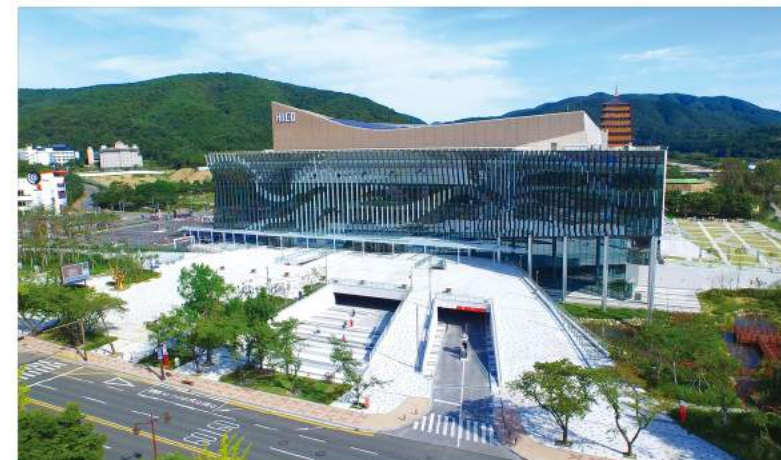
Gyeongju Hwabaek International Convention Center [Culture Facility] Total Ground Area 31,259m 2 , B1-4F, Large Conference Room with Seating Capacity of 3,420, Other Amenities
